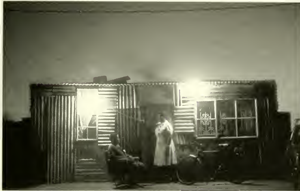
Above: Corrugated iron sheets are often used for make-do homes in squatter settlements.
